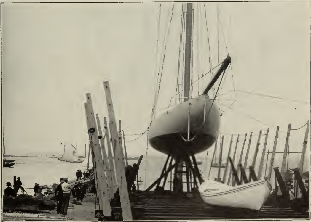
RELIANCE ON THE WAYS, SHOWING UNDERBODY AND FIN KEEL.
